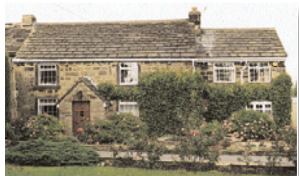
Abbey House, converted farmhouse
