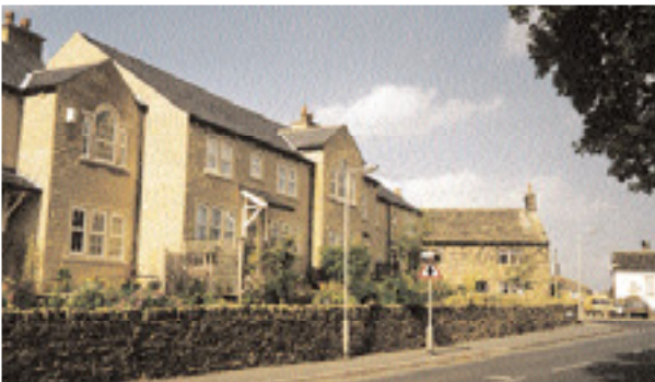
Old Forge Mews, former garage site
