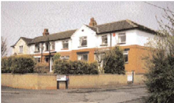
Former council houses
