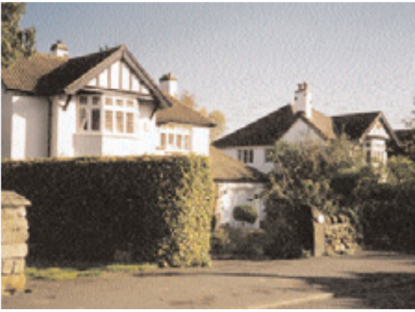
Breary Lane, substantial 1930s houses
